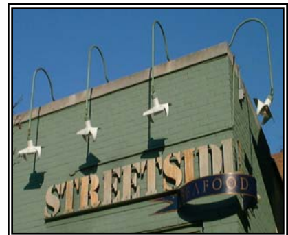
Front Lit Wall Sign Gooseneck lights
